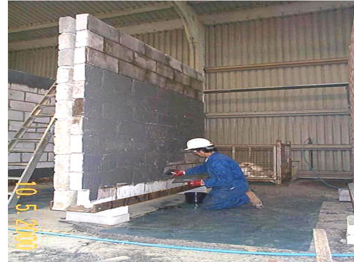
Composite reinforced masonry wall
